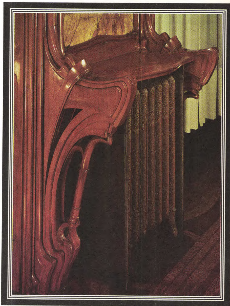
The climate control is total and self-regulating from the top to the ground floor. In the dining room it is governed by two intake-radiator units and assisted by one exhaust stack, a second air passage, four regulatory screens and one auxiliary gas heater.
